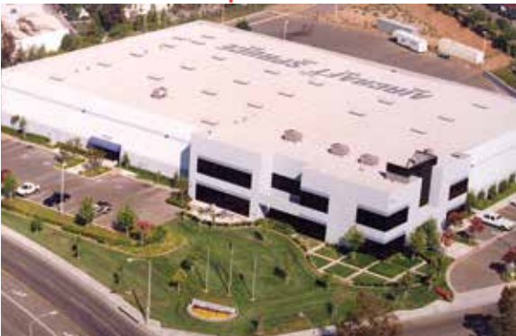
Present Home of Aircraft Spruce West (225 Airport Circle, Corona, CA.)
